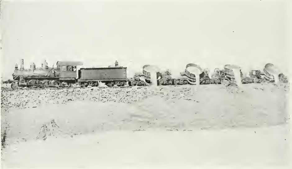
Fig. 76—Pouring Slag on Dump, Canadian Copper Company, Copper Cliff, Ontario.
